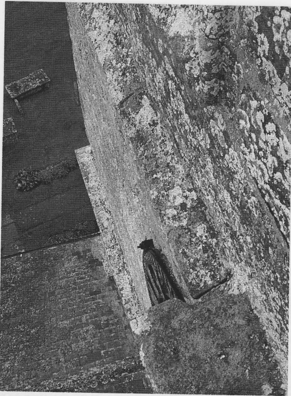
Tower east elevation – open joints in parapet string course.
