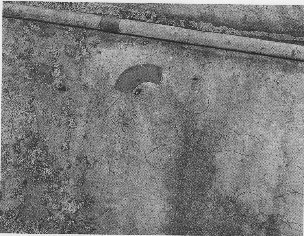
Graffiti on tower roof leadwork and previous patch repair
