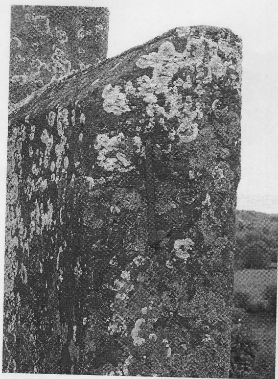
Tower parapet – iron cramp and fractured stone.
