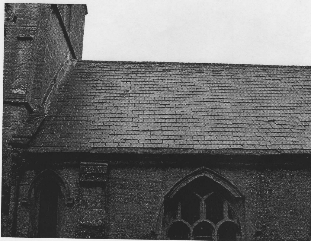
Nave north slope -- slipped/missing slates.
