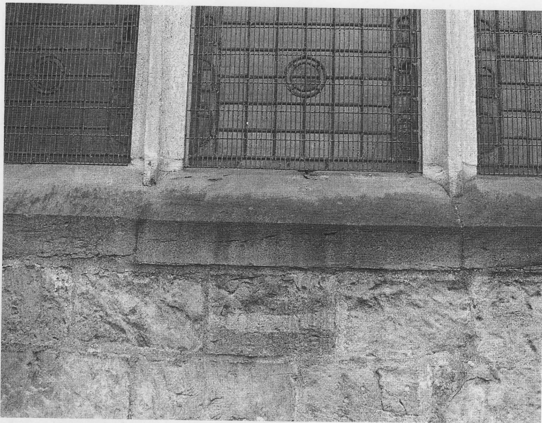
Staining from rusting window guards.
