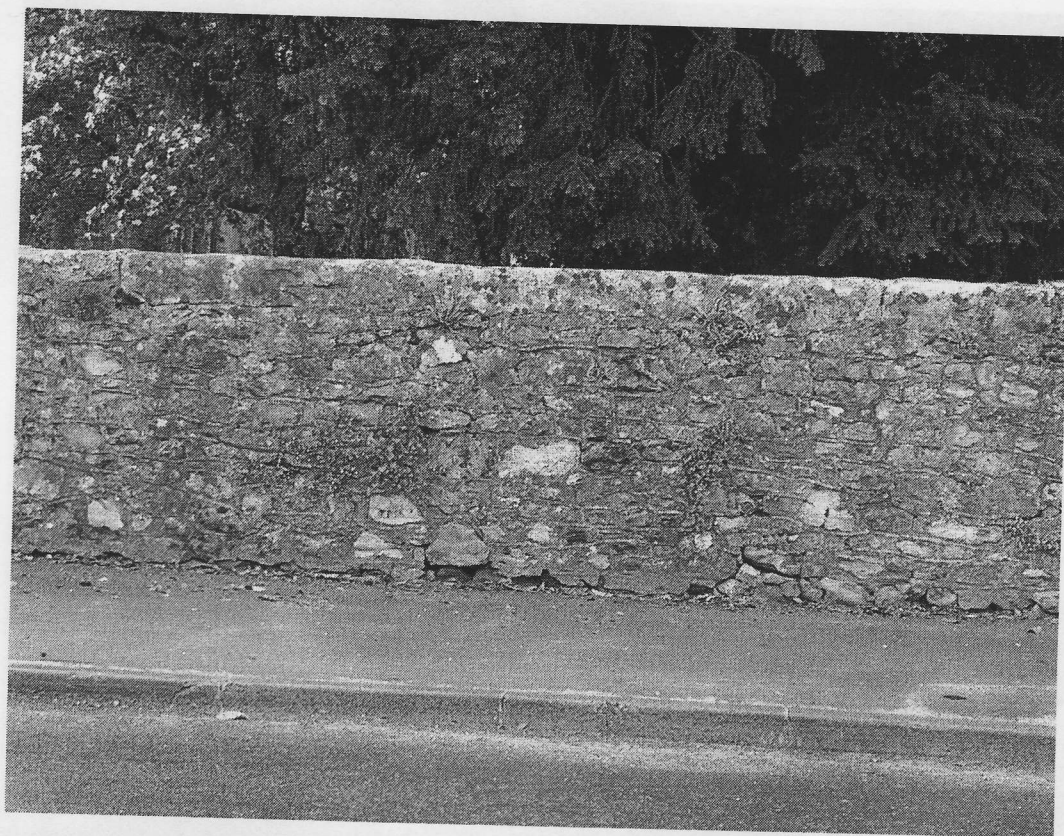
East boundary wall – open joints, particularly at low level.
