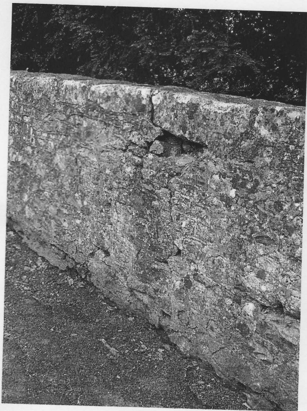
North boundary wall – loose/missing stonework and open joints.
