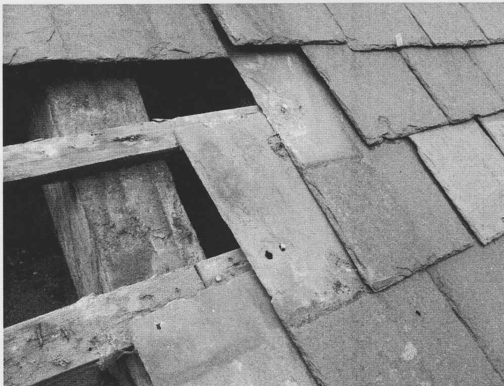
Slates on nave roof fixed to large battens. Poor nail fixing and reholing of slates (for reuse) visible.
