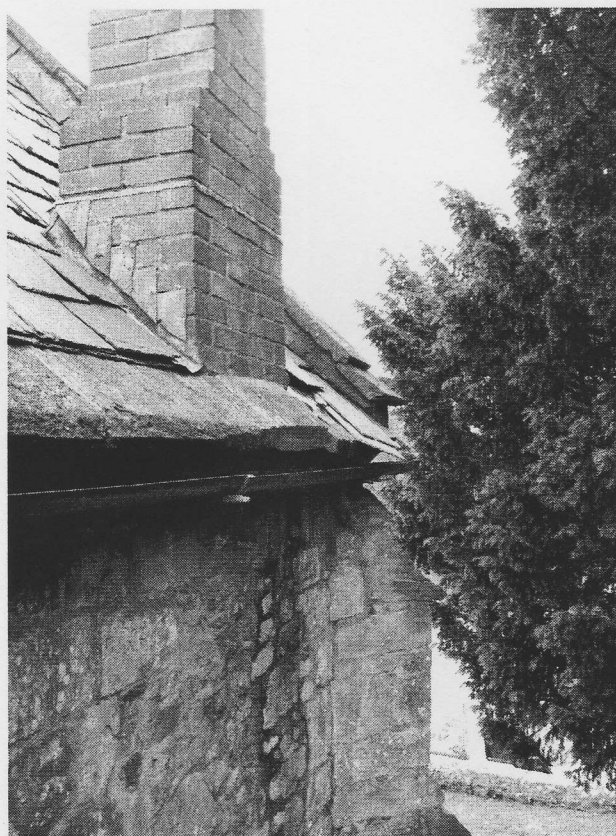
Slipped slates (to right of chimney) at west end of north roof slope. Lead tingles visible above chimney, forming new fixings for previously slipped slates. Water staining visible on wall where roof coverings have failed.
