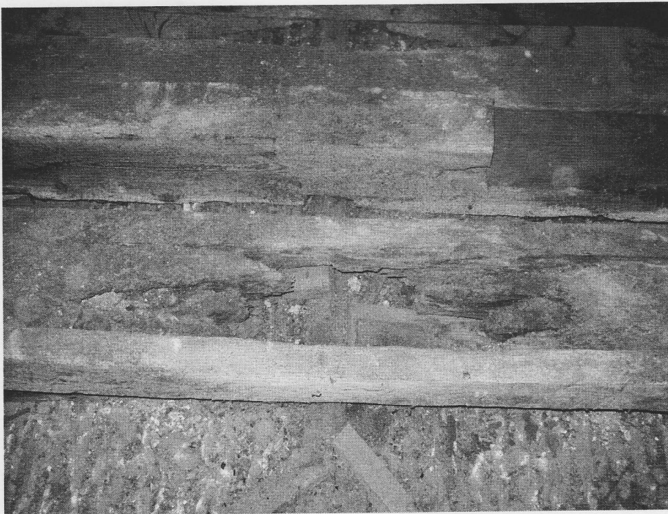
Severe decay to elements of the roof structure previously repaired.
